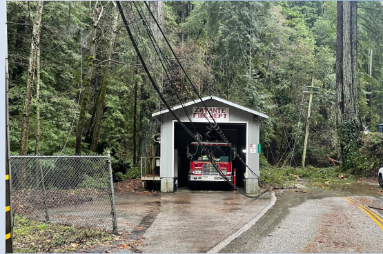
Zayante Fire Station #2
